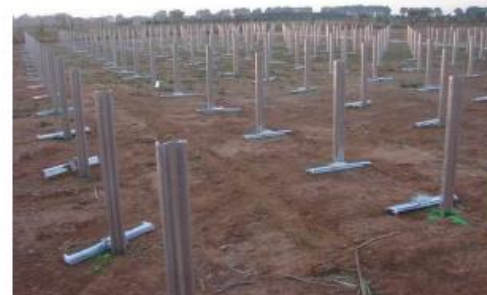
Aspect des supports
